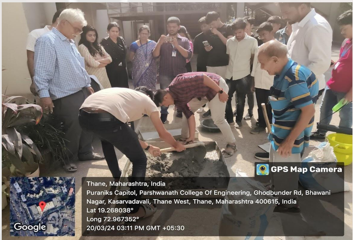
Students Preparing Mortar
