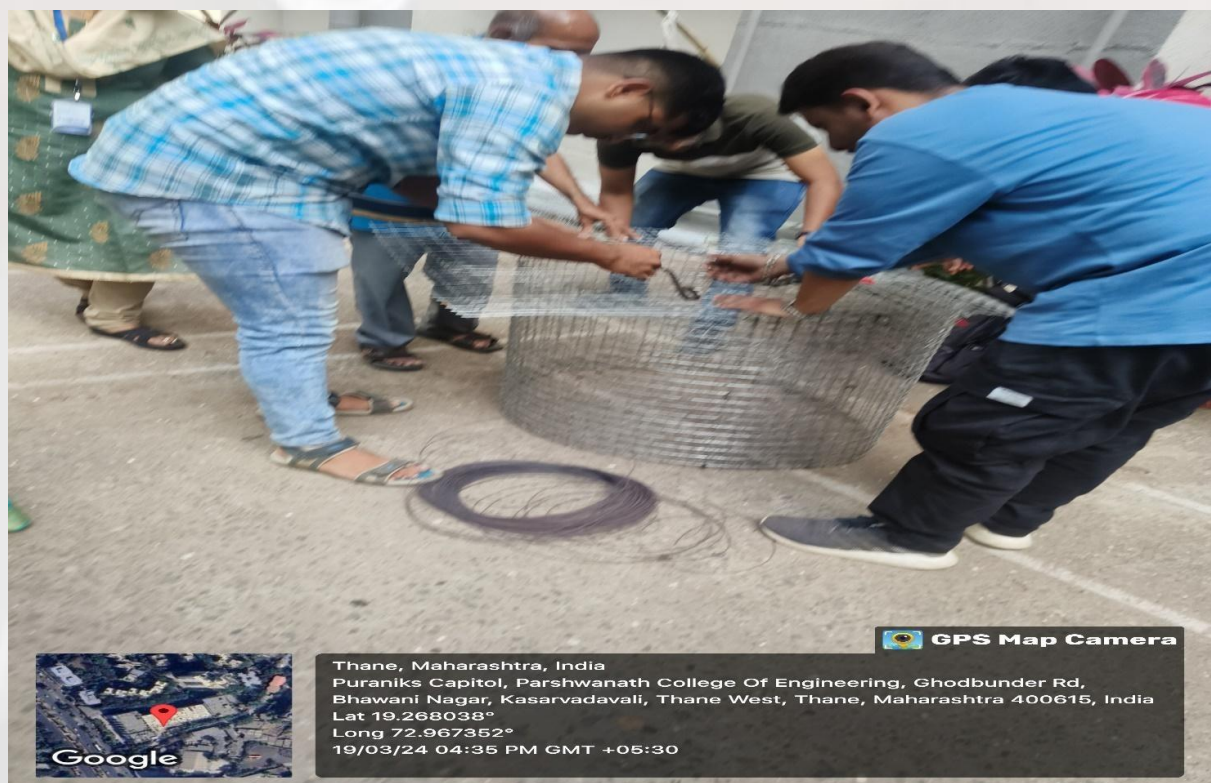
Students Binding the Weld and Chicken Mesh for Ferrocement Tank Skeleton
