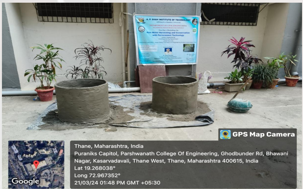
Ready Ferrocement Tanks
