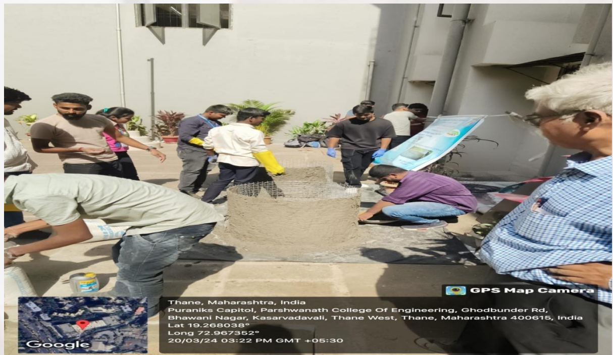
Mortar Filling on Skeleton
