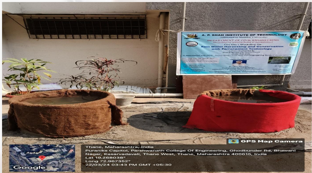
Tank Curing in progress
